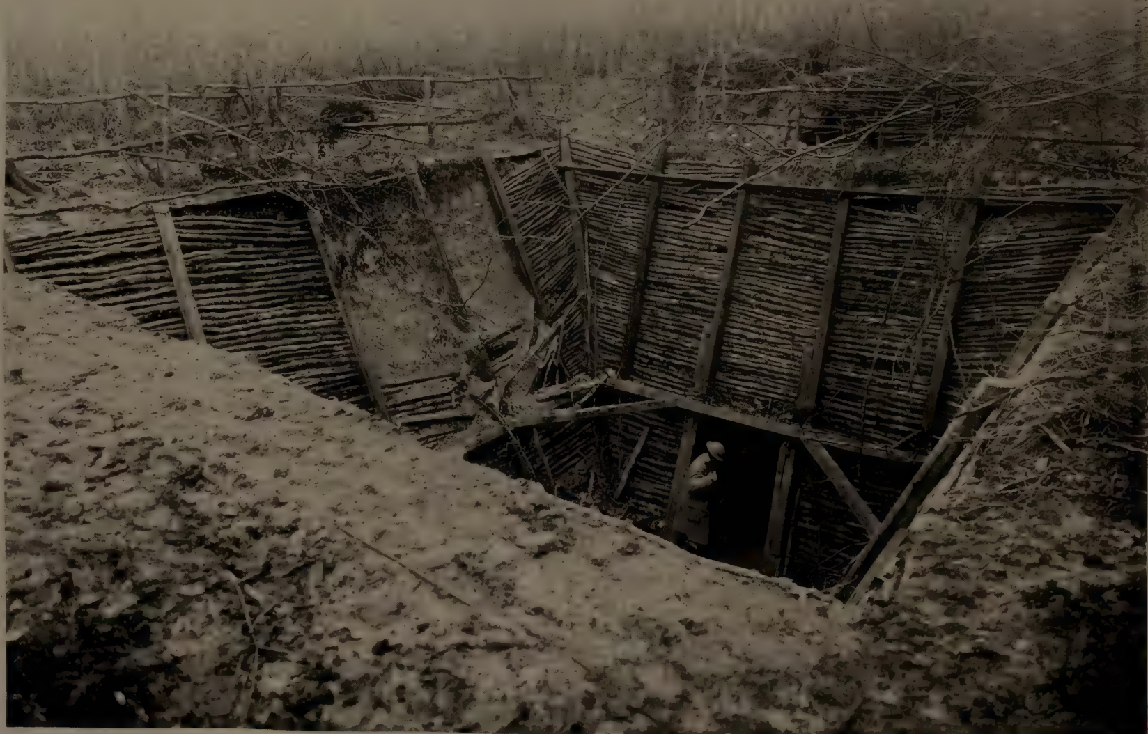
One of Eight Entrances to Dug-Out, "Bois de Chaume," Bottom of Dug-Out two flights of Stairs below where Soldier is standing, or about Sixty-five ft., Accomodating about fifteen hundred Men.
